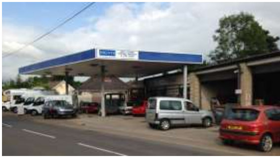
Figure 11 F E Brent and Sons Garage
